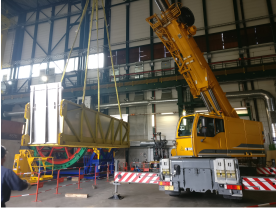
Figure 4.5: A crane in CMS-S being used to transport a large box containing the demonstrator detector, readying it to be lowered down the main shaft.
