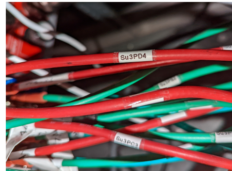
Figure 5.73: Each SHV cable is labeled with the code according to Figure 5.61.
