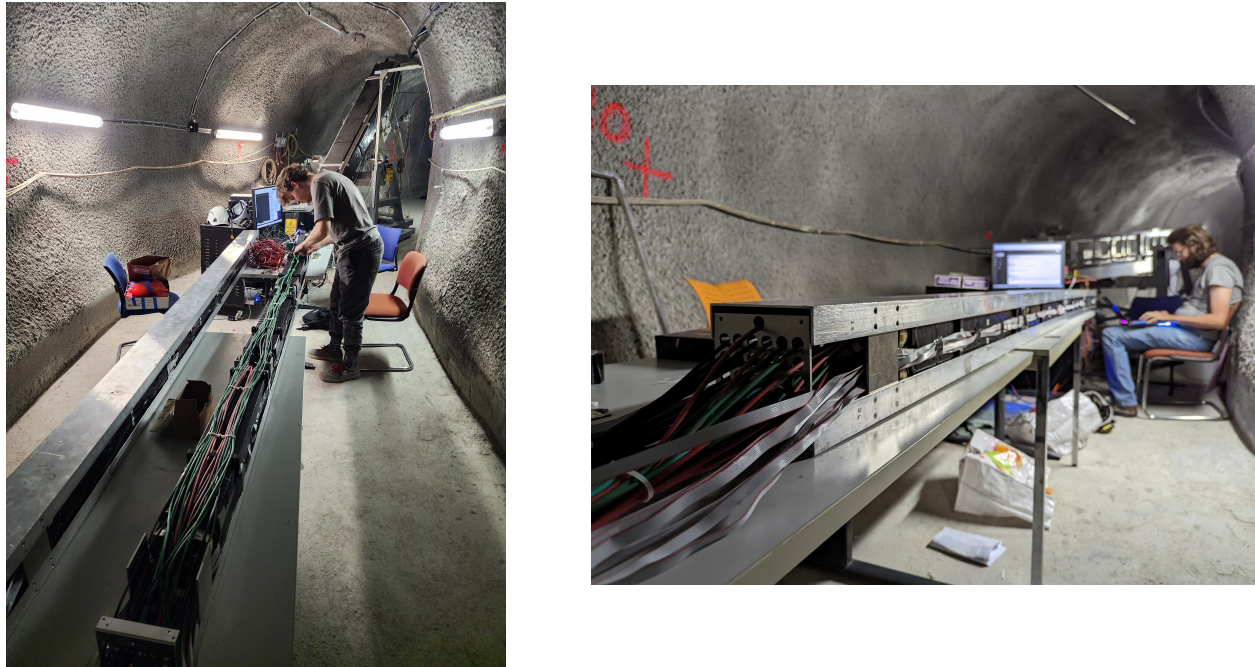
Figure 5.17: A fully assembled, cabled supermodule. HV and signal BNC cables are laid across the top tray of the supermodule, while low voltage ribbon cables weaved through the side. (Left) UCD graduate student Jacob Steenis working on the supermodule. (Right) The author, analyzing data after assembly.
